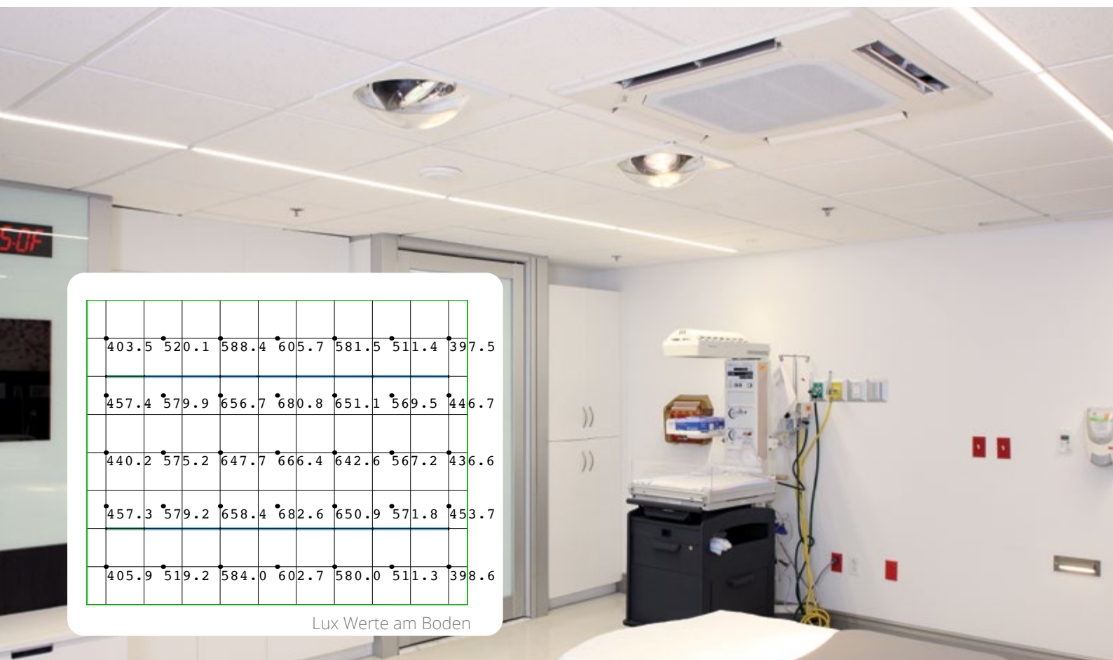
Springhill Medical Center – Mobile, AL AMA Lighting
